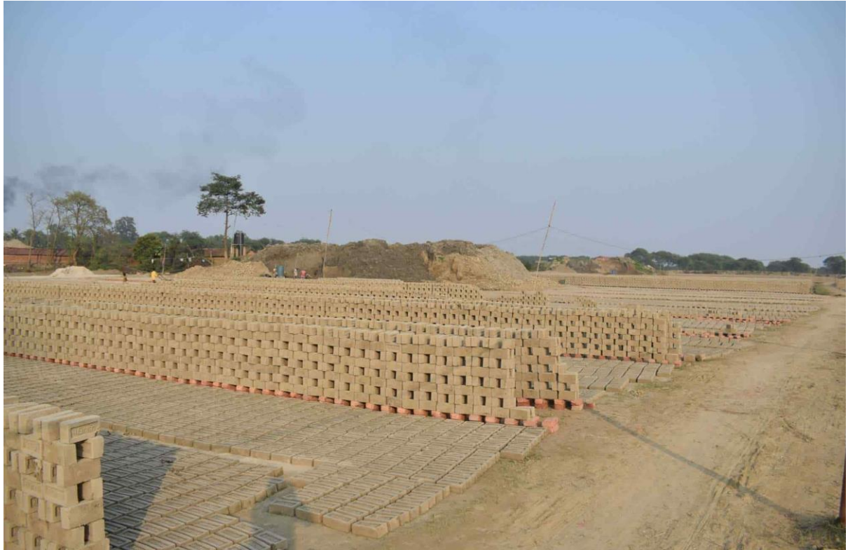
Image No103: New Tribeni Bricks, Bally
